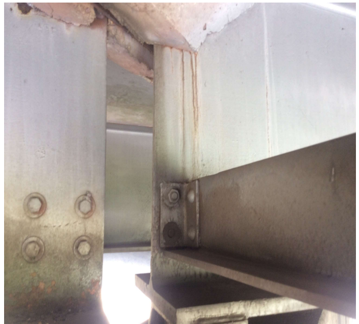
PHOTO 2 Description Bent 2 girder 3 has 2 sheared bolts.
