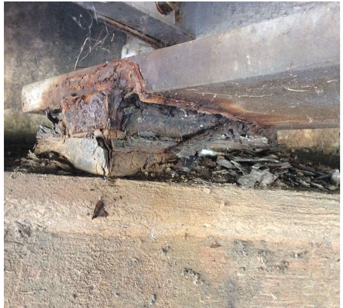
PHOTO 2 Description Bent 4 bearing 2, laminating/pack rust.
