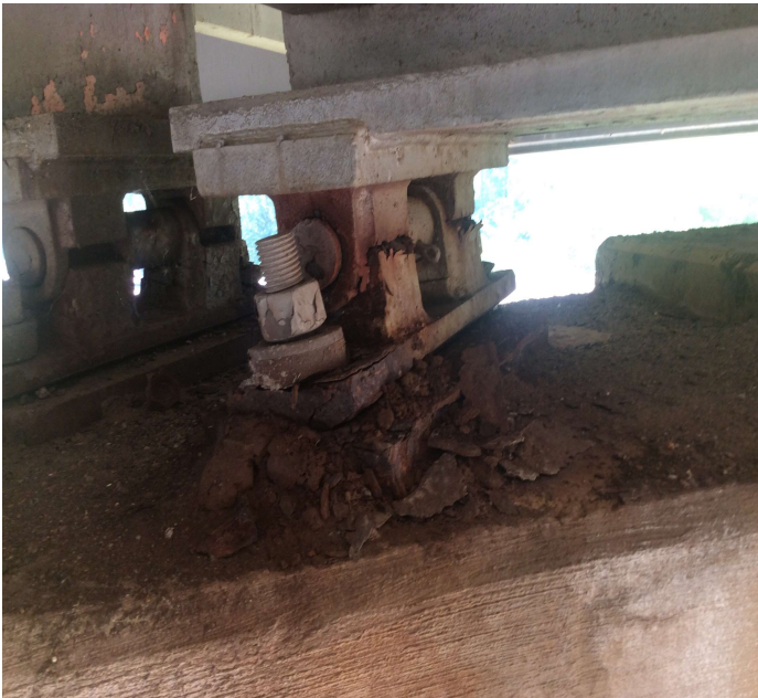
PHOTO 1 Description Bent 3 girder 6 bearing has laminating/pack rust.
