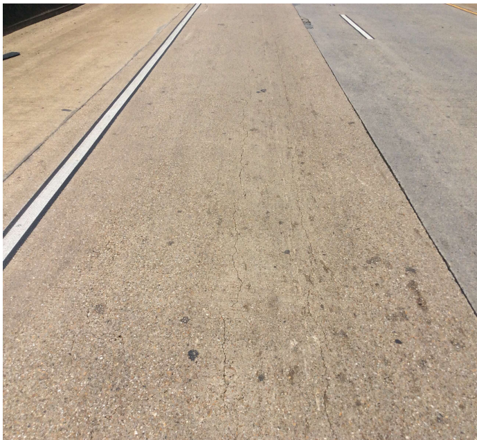
PHOTO 1 Description Span 3 longitudinal cracking in deck.
