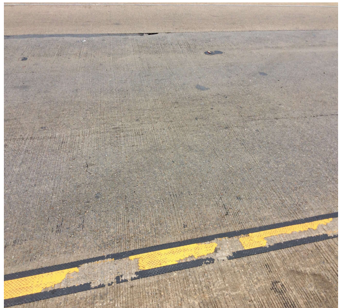
PHOTO 2 Description Transverse cracking span 3.
