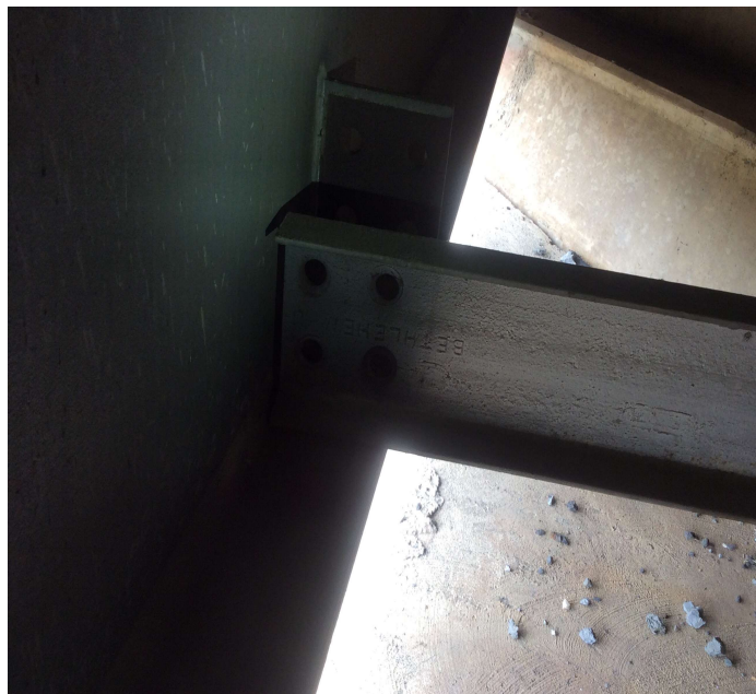
PHOTO 1 Description First diaphragm at bent 1 between girders 6 and 7 has loose and missing bolts.
