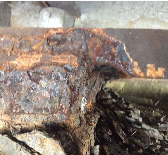
PHOTO 1 Description Bent 4 girder 2 has 5/16" section loss to bottom of bottom flange.
