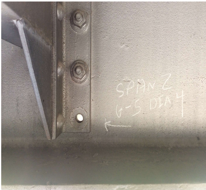
PHOTO 1 Description Span 2 girder 5 has a missing bolt in bottom of diaphragm connection.
