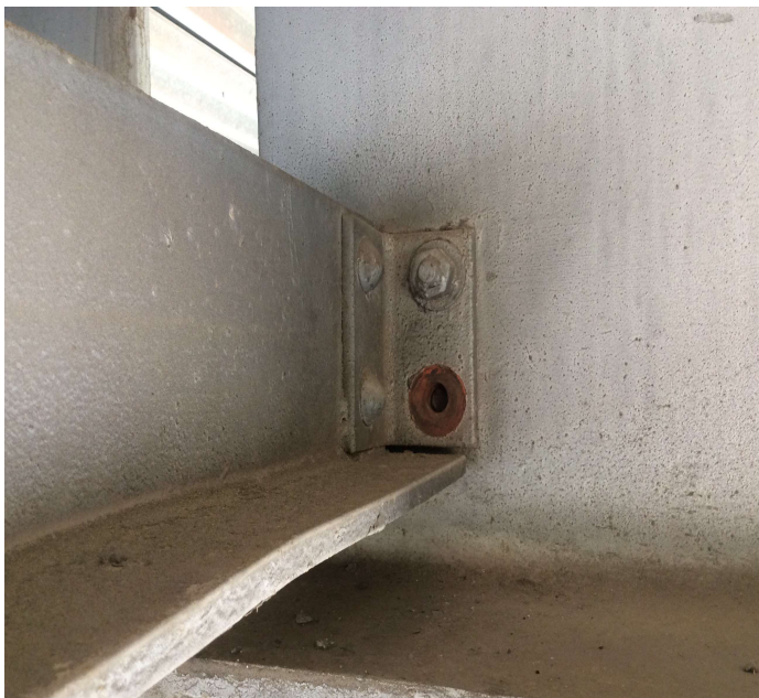
PHOTO 3 Description Bent 3 girder 6 sheared bolt in diaphragm connection.
