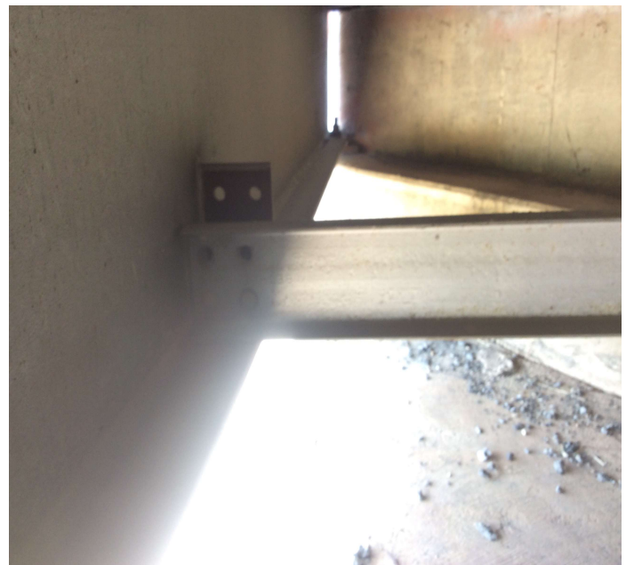
PHOTO 2 Description Span 1 girder 7 diaphragm 1 is sitting on bottom flange, all 4 bolts are loose on girder 6.
